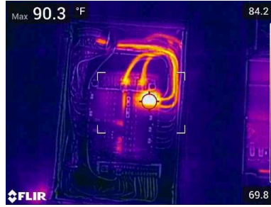
Normal temperature range observed at the time of the inspection
