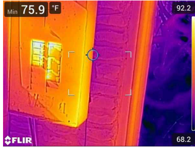
Normal temperature range observed at the time of the inspection
