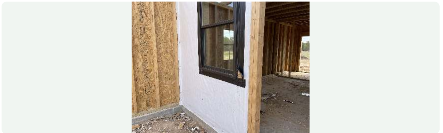
Front bedroom window - wider view
