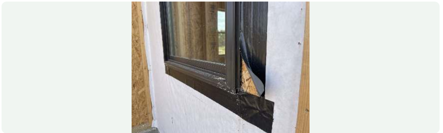
Front bedroom window - detail
